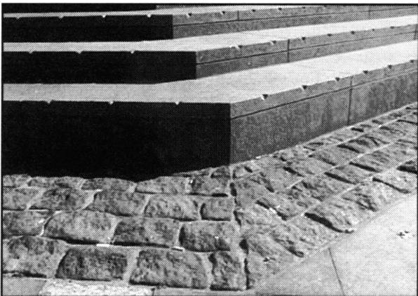
Divots and cobblestone: the new Ferry Plaza appears public by virtue of the invisibility of its deterrents.
